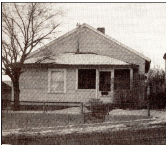
1909-1911--"D" Street, Rock Springs, Wyoming
