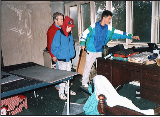
Jim, Spence and me facing the damage
