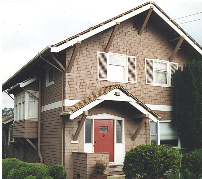
Myrl Owen's Home at 22 Nace Street (Gordon & Alice lived in downstairs apartment)
